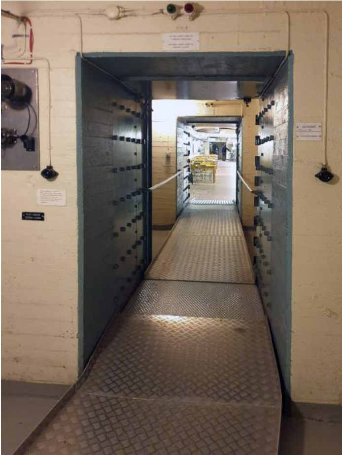
Internal blast door in Storåberget .
