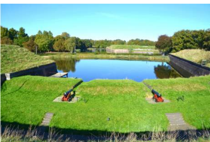
Fig. 30: View from the Turfpoort bastion (fortress museum) across the cannon yard to the access road to Naarden fortress
