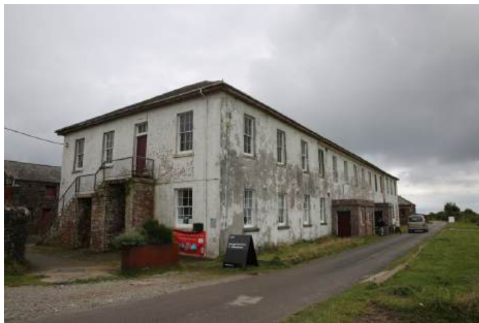
Fig. 7: Maker Barracks completed in 1808. (Photo: Nick Dougan)
