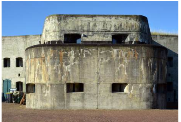
Fig. 34 Two-storey traditor casemate in the gorge of fort near Hoofddorp. The fort now serves as a restaurant and theatre.
