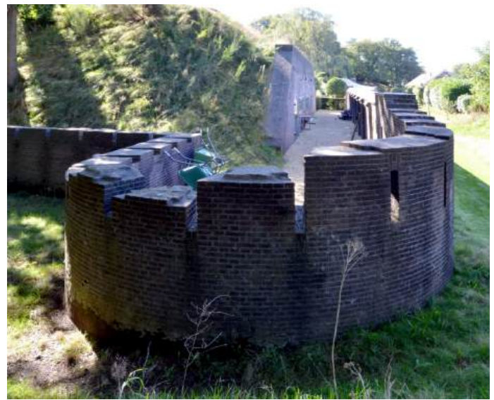
Fig. 32: Thoroughly renovated Carnot wall at Works IV in Bussum
