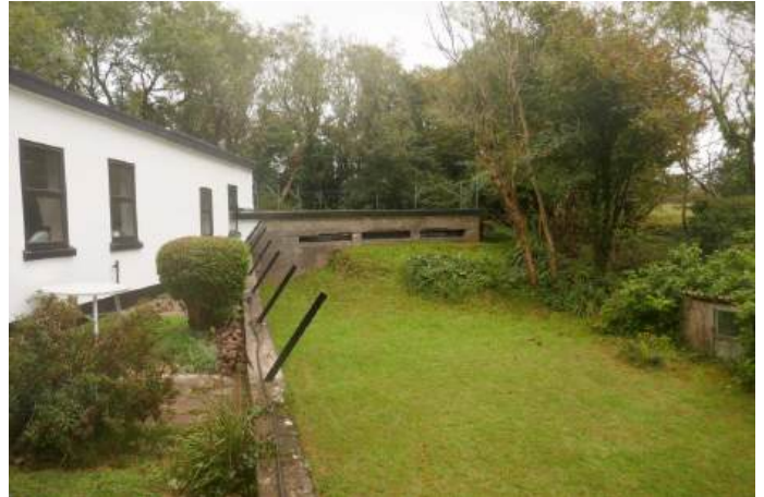
Fig. 10: Hawkins Battery; looking along the line of the ditch to the eastern blockhouse. 1900 fitters shop to the left. (Photo: David Clarke)
