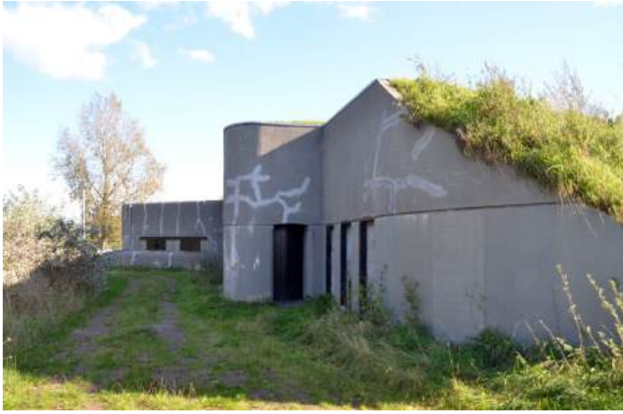
Fig. 28: Renovated rear with traditor casemate of the fort near Aalsmeer
