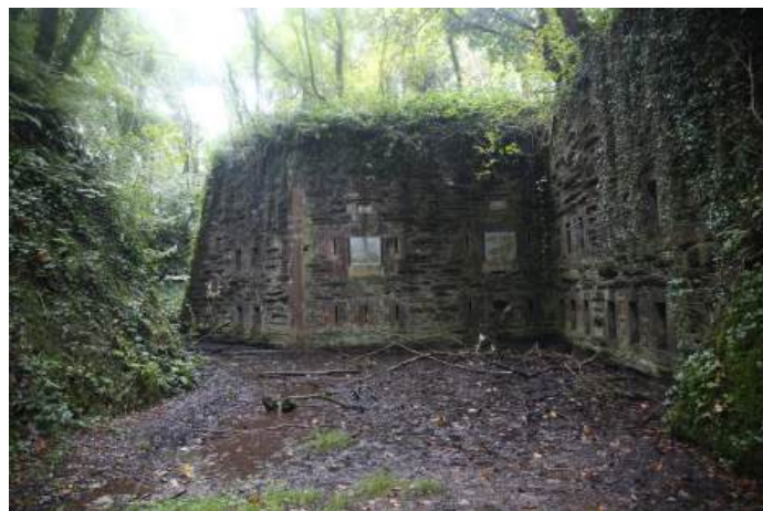
Fig. 7: Woodland Fort; northeast caponier from the ditch. (Photo: Nick Dougan)
