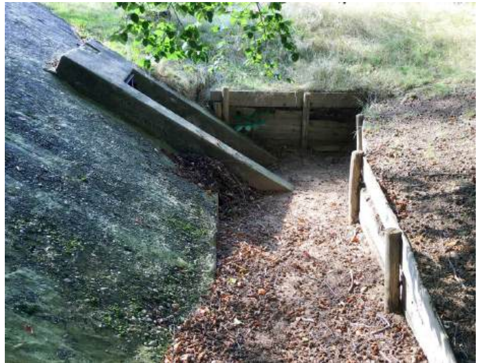
Fig. 33: An uncovered entrance to an object in the 'Franse Kamp' bunker complex in Bussum
