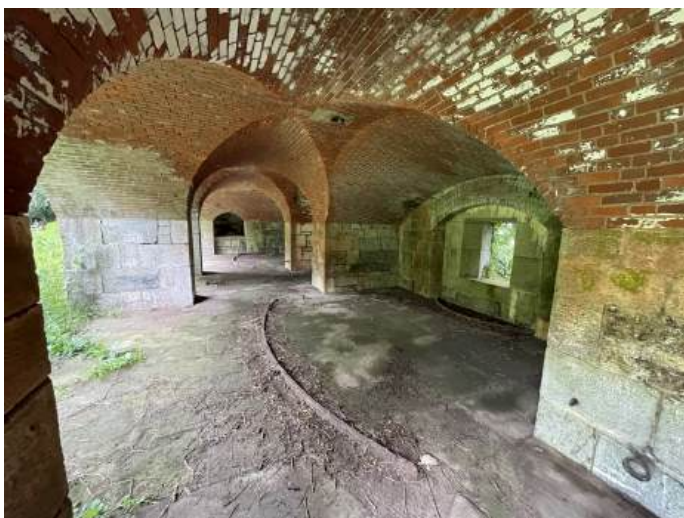
Fig. 3: Scraesdon Fort; Haxo Casemates in the lower level. (Photo: David Clarke)
