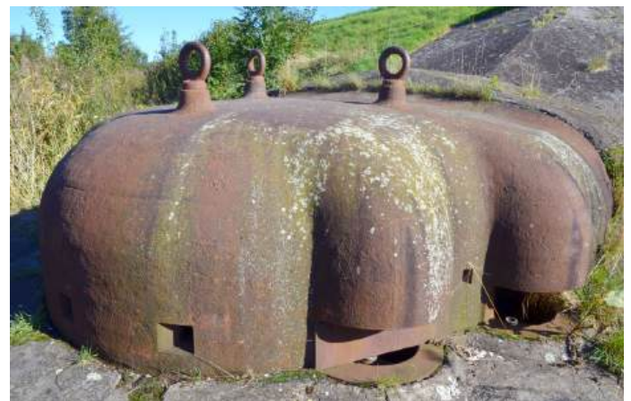
Fig. 26: Armoured bell for small arms at the end of the fort's poterne near Hoofddorp
