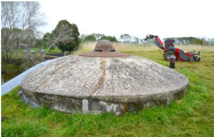
Fig. 21: Observer's bell against the background of an automatically operating lawnmower on the roof of Fort Waver-Amstel
