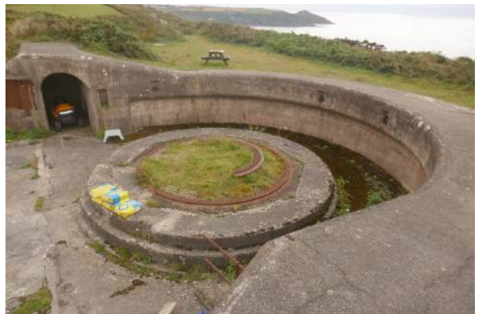
Fig. 4: Whitesand Bay Battery; emplacement for 12.5 inch RML on 'small port' carriage. (Photo: David Clarke)
