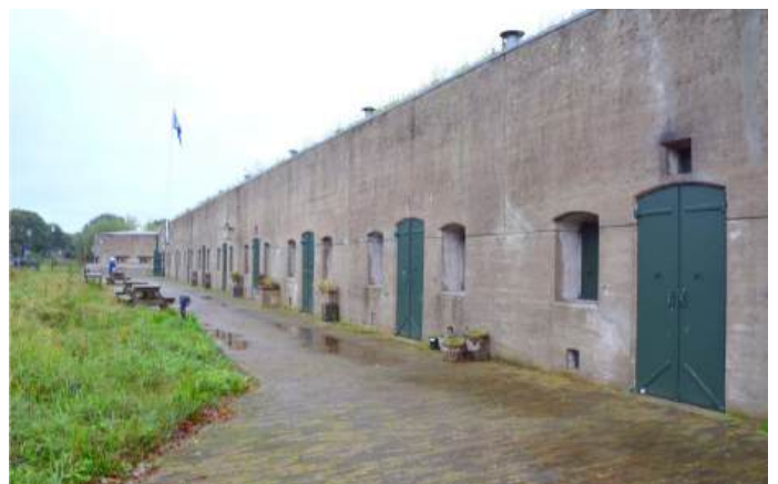
Fig. 19: Rear of the main building with traditor casemate in the background of the fort on the Drecht
